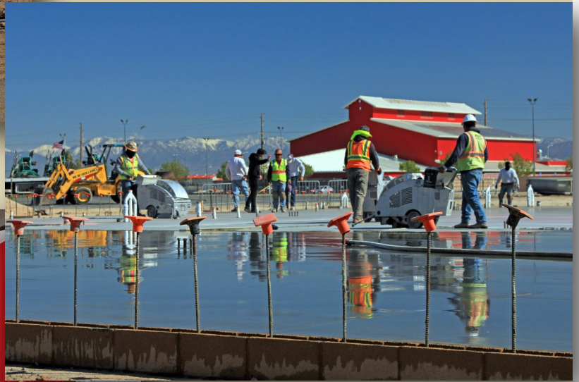
Toneman Development Corporation, our General Contractor, places the concrete for the foundation and floor.
